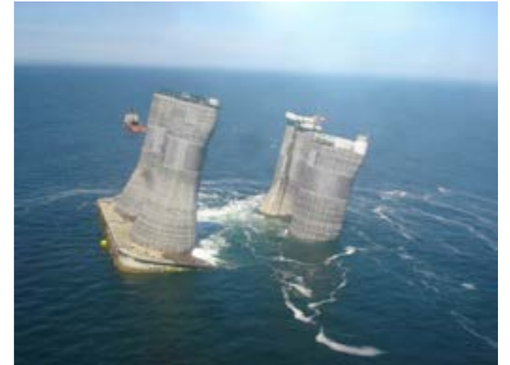
GBS installation at field (Source: Kvaerner)
