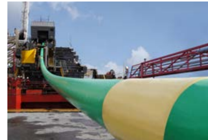
Goliat Platform (Source: Bredero Shaw)
