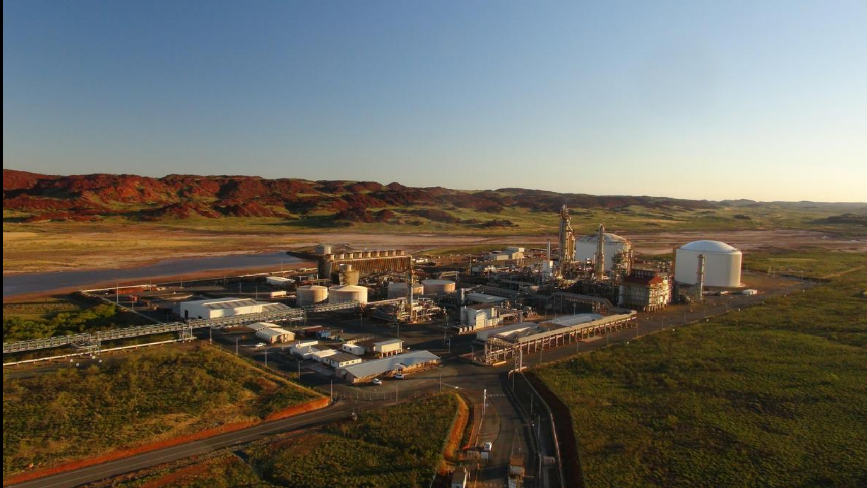
Yara Pilbara Ammonia Plant
