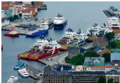
Shore power solution
